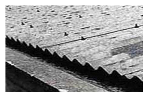
Asbestos cement products, which can be fully or semi-compressed into flat or corrugated sheets. Corrugated sheets are largely used as roofing and wall cladding. Other asbestos cement products include gutters, rainwater pipes and water tanks.
