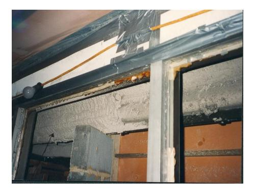
Sprayed asbestos and asbestos loose packing - generally used as fire breaks in ceiling voids.
